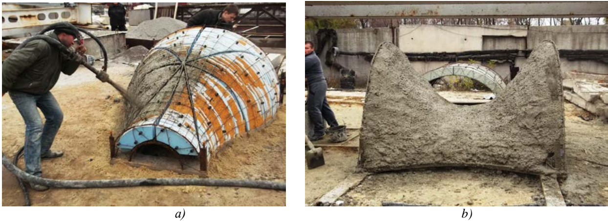
Figure 1: The process of wet gunned shells with a working nozzle with a ring nozzle (a) and a finished reinforced concrete shell (b)
