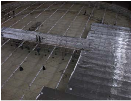
Picture 2. Installation of aluminum floating membrane in the storage tank
