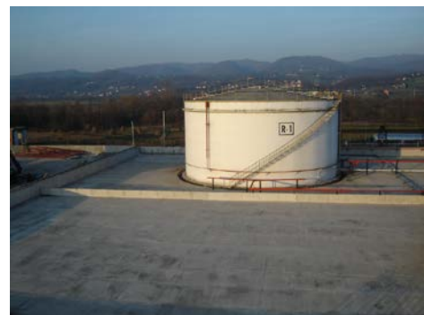
Figure 1. Storage tank for oil derivatives
