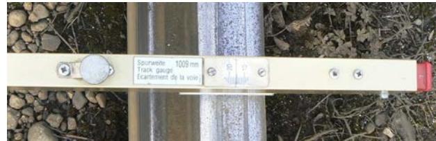
Picture 2: Track - measurement of track gauge.
