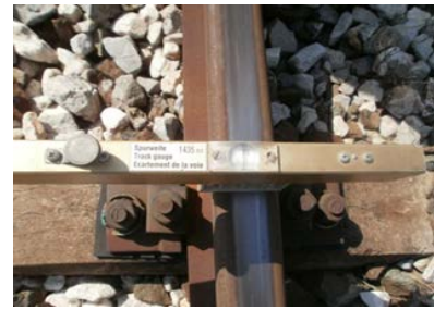
Figure 5: Control of the track gauge and superelevation
